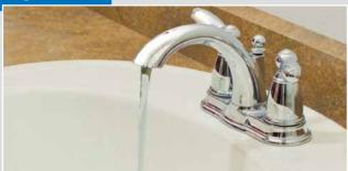
RUN COLD WATER AT FULL VOLUME FOR AT LEAST 2 MINUTES. This will ensure that all of the bleach has been rinsed from the faucet and that the water you are sampling has not been sitting in the pipes or tanks for a long time.
